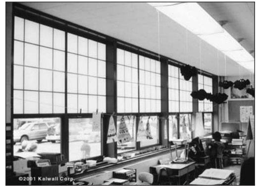
Figure 6.16: An example of a Kalwall glazing used in an elementary school in Rochester, New Hampshire. This is the R-10 translucent glazing material, a double surface fiberglass with insulation between the fiberglass sheets. The view is from the inside of the building, so that actual light levels are shown. (Photo from www.kalwall.com )
