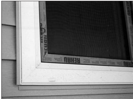
Figure 6.22: This window frame sits outside the insulated wall.
