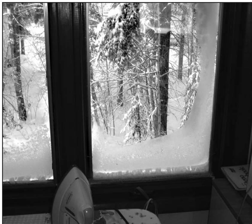
Figure 6.12: Frost has built up between the storm window and the main window. It will eventually melt and cause water damage.
