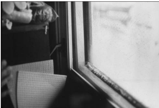
Figure 6.14: Ice accumulation from condensation on the very bottom of a window: the coldest place on any window surface.
