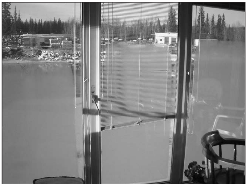
Figure 6.13: There is condensation on the outside of these windows, but the edge effect and a roof overhang make the edges and the top of the windows warm enough to be frost-free.
