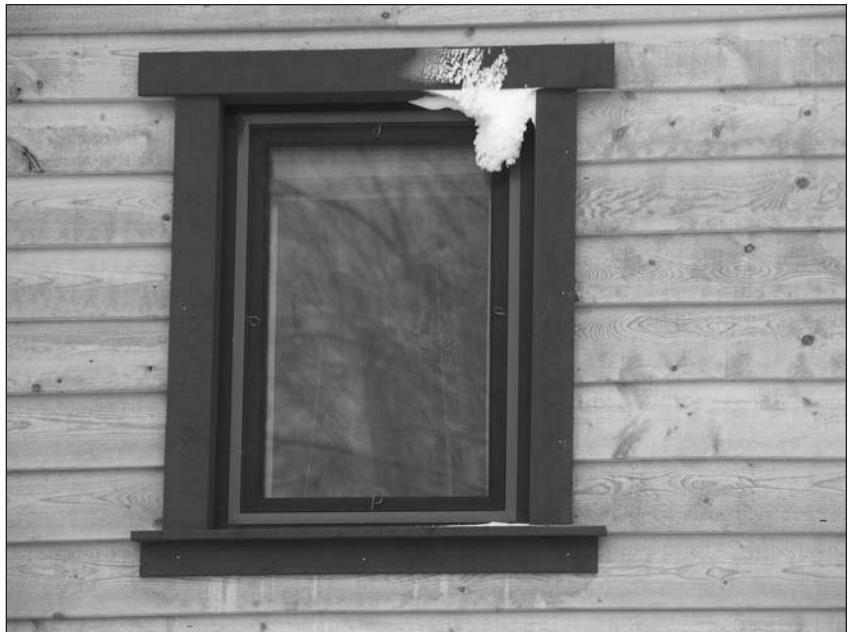
Figure 6.19: This frost on a second-story window is the result of air being pushed out by the stack effect through a poorly installed seal around the window.
