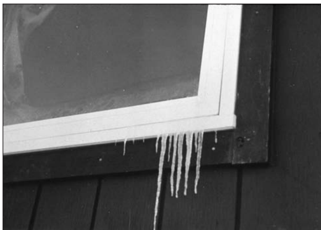
Figure 6.1: This window is weeping moisture because condensation is thawing inside, running out the weep holes, and refreezing outside.
