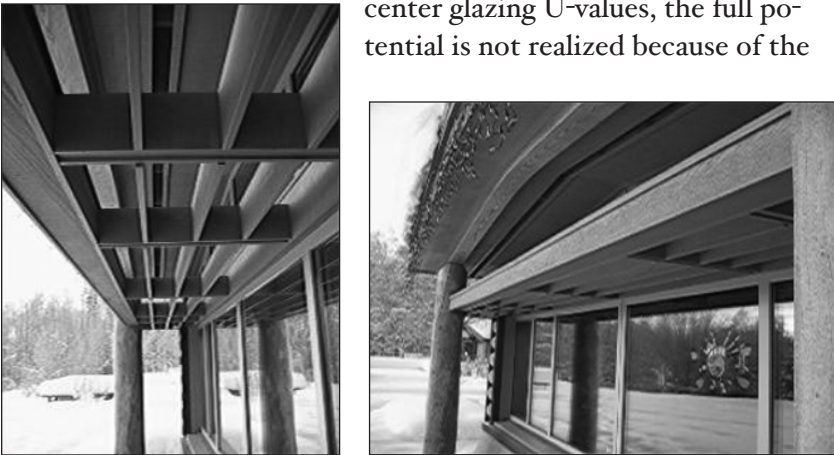
Figure 6.20: Two views of the very well designed architectural shading devices used on the home of the University of Alaska president. The left photo is a view from the front and the right photo is a view looking upward from below the shades. These devices have many advantages: they are in a fixed position, so they don't need to be moved seasonally; they are not solid so they easily allow shedding of snow, and because they are not solid, they allow indirect light to pass through them even when the direct light is shaded.
