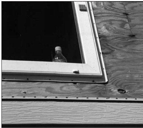
Figure 6.21: Mounting a window using the nailing fin is not a good idea.
