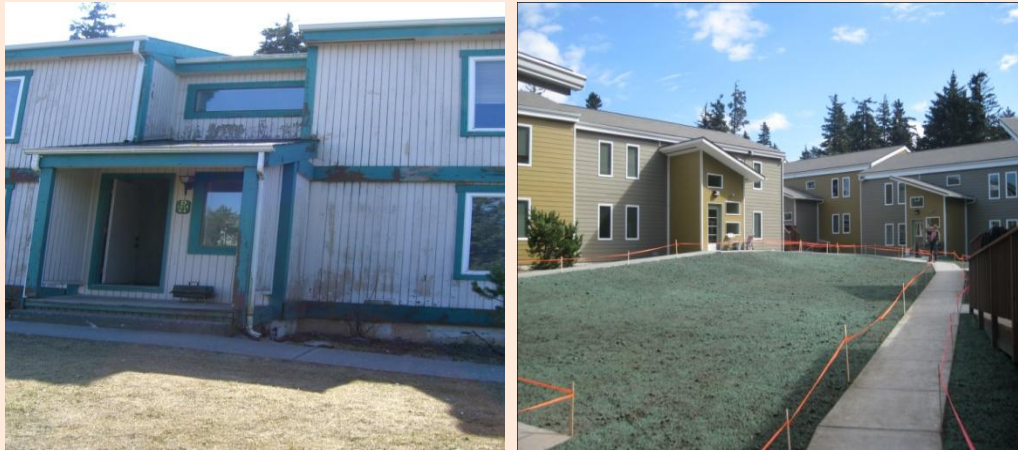
Renovation: Before & After (Kodiak)
