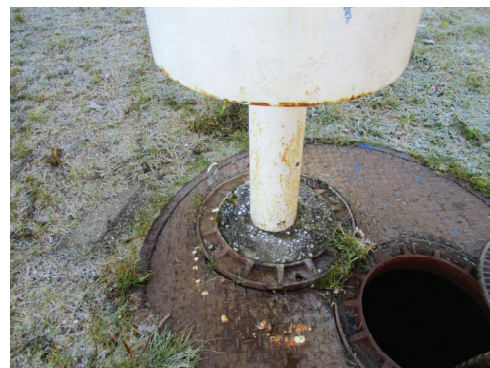
Replacement sump inside old sump
