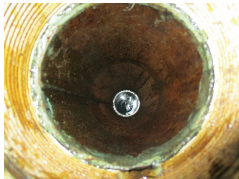
Fuel fill overfill device
