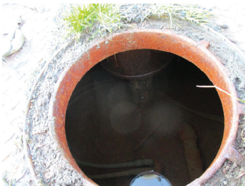
Piping sump full of water
