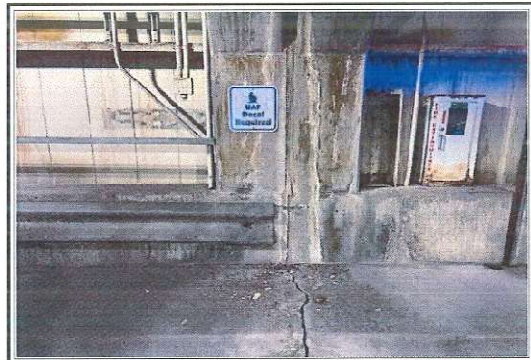
Damage - crack in concrete
