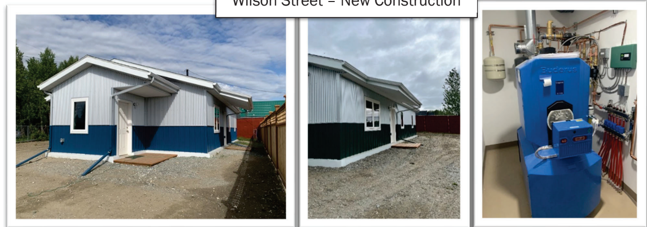
Wilson Street – New Construction
