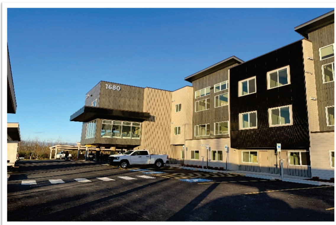
Aspen House by Wasilla Area Seniors. 40 units newly constructed in Wasilla.
