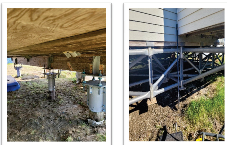
Foundation Leveling for Nome and Bethel housing developments
