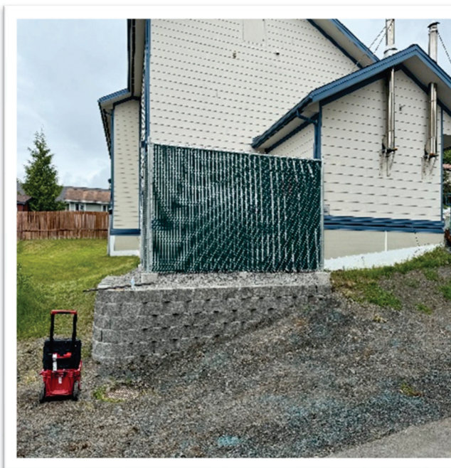
Above-Ground Storage Fuel Tank and Enclosed Surround – Sitka
