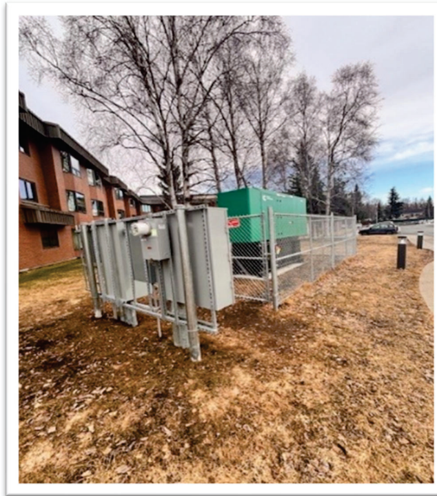
Auxiliary Generator Installation for Chugach Manor – Anchorage
