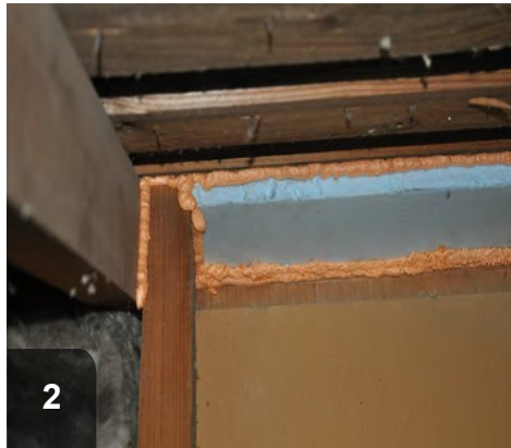
2 Top plate has been sealed to adjacent framing
