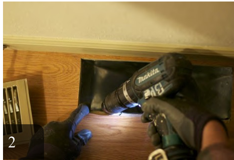
2 Use fasteners to close gaps before applying mastic
