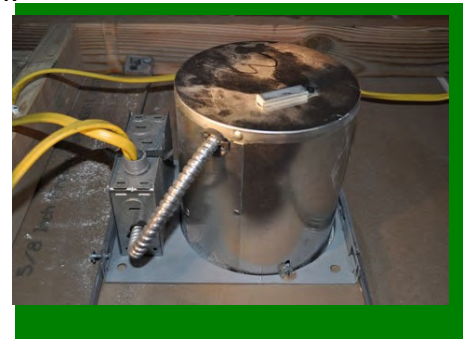
Airtight IC rated recessed light
