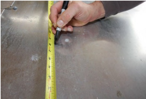
Determine and mark truss locations on roof, and choose method of access. Avoid drilling or sawing into trusses
