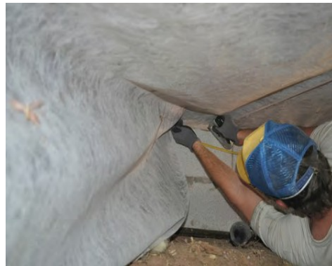
Secure netting across sills to prevent leakage of insulation
