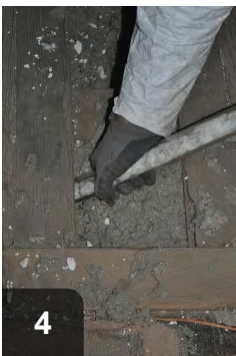
4 Where flooring cannot be removed, verify insulation is meeting R-value goal
