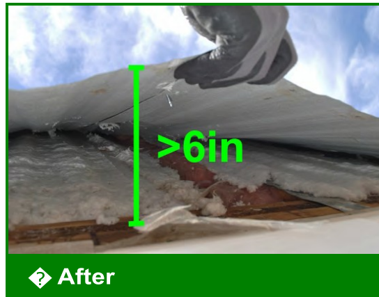
Remove enough fasteners to create at least a 6in gap without damaging siding
