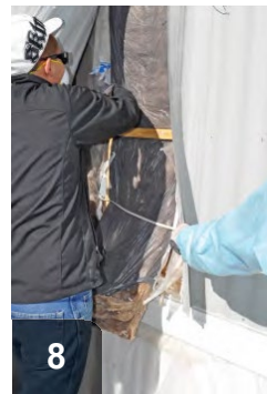
8 Tuck bottom of batt behind bottom belt rail. If longer than cavity, cut to within 1" longer, roll and tuck into cavity
