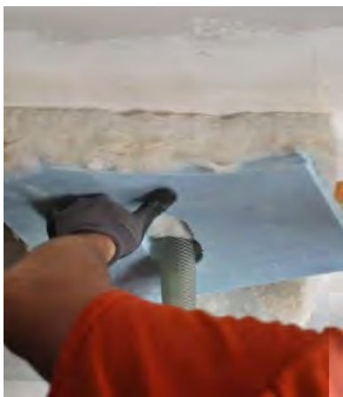
Blow insulation into cavities to density appropriate for chosen material
