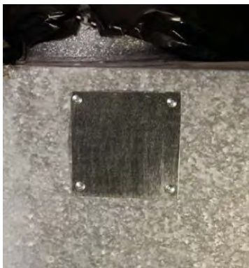
Install rigid duct support material that at least 1 inch larger than the hole.
