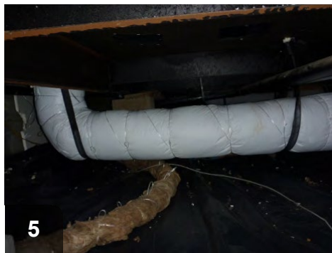
5 Insulate and support crossover duct
