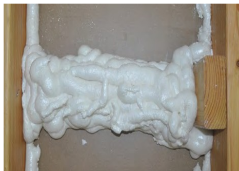
Option 2: Bridge cavities with spray foam
