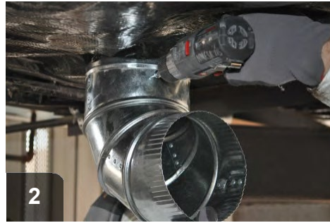
2 Fasten elbow in place with at least three evenly-spaced fasteners
