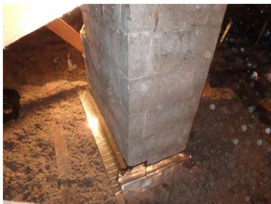
Only construct dam after sealing has been completed properly.
