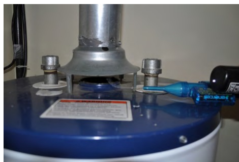
Assure draft using a smoke pencil, mirror, or lighter,
