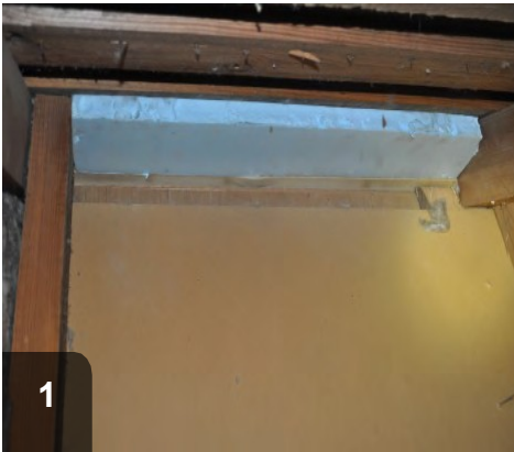
1 Top plate has been cut and fit to size
