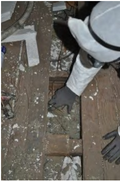
Check cavity for electrical junctions and penetrations
