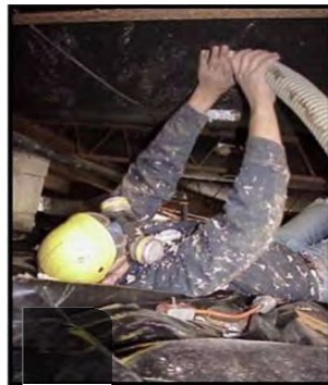
Loose fill insulation is blown into mobile home belly cavity.
