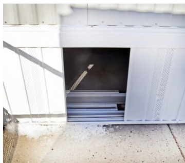
If skirting overlaps siding, remove skirting
