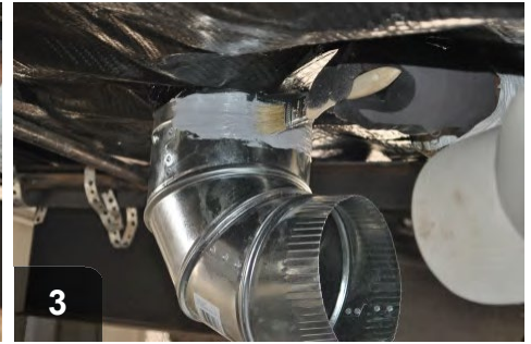
3 Apply mastic at all metal-to-metal connections
