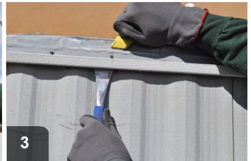
Cut through putty tape and pry J-channel away from roof seam
