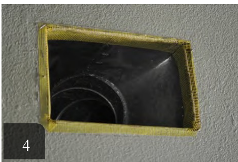
4 Cut mesh to fit around duct boot and cover gaps
