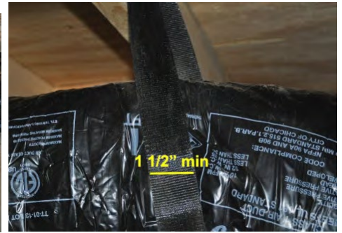
Durable strap should be at least 1 1/2 inches wide
