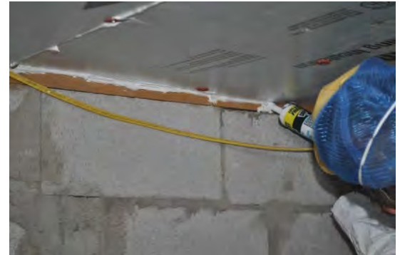
Once rigid barrier is sealed, insulation can be blown in
