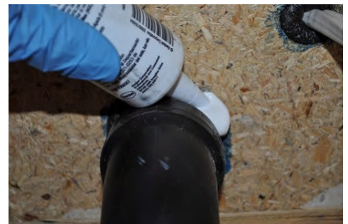
Caulk smaller gaps and to hold backer rod in place
