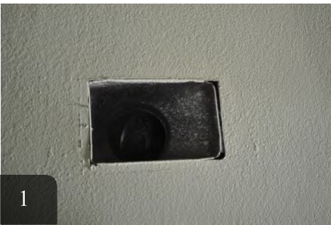
1 Remove grill to expose duct boot and gaps
