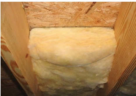
Batt must be in contact with subfloor without voids, gaps or being compressed
