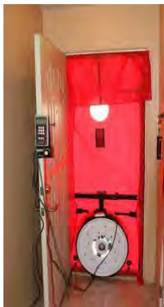
Set up blower door and depressurize bonus room to -50pa wrt outside
