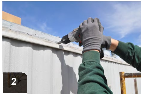
Remove fasteners from the J-channel
