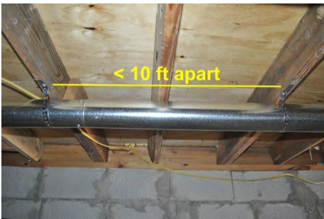
Metal ducts should be supported every 10 feet or less with straps or wire
