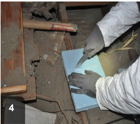
4 Bottom plate is cut to size
