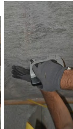
Keep netting taut while stapling to prevent wrinkles and leakage
