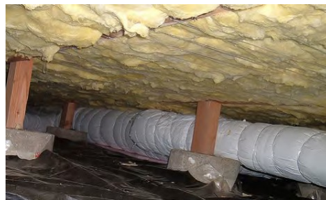
Twine fastened across bays in a zig-zag pattern
