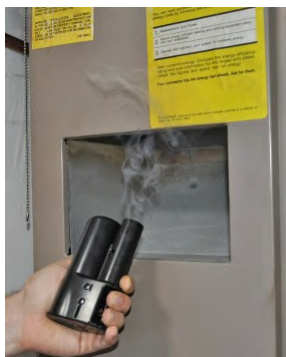
Complete spillage testing on all atmospheric combustion appliances
