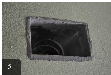
5 Apply mastic over tape to create heat resistant, durable bond, allow to dry
