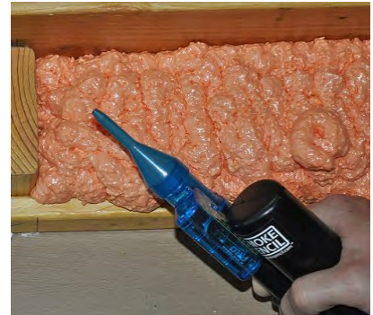
Whatever option chosen, test to verify no air leakage
