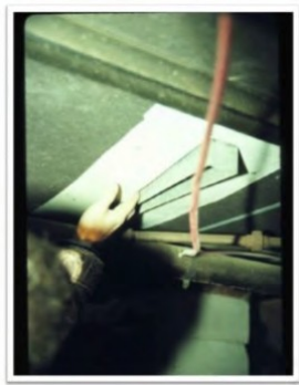
Maintain all combustion air intake openings when patching belly material.
