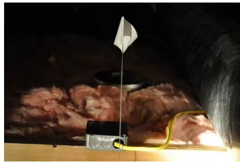
Flag and install covers on electrical junctions
