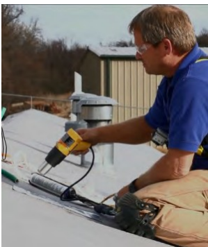
Use a heat gun to make the adhesive pliable to get the best possible seal.
