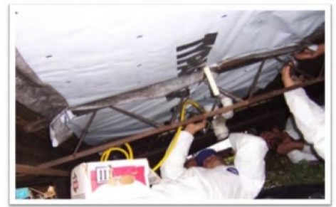
Workers install new material where rodent barrier is missing
