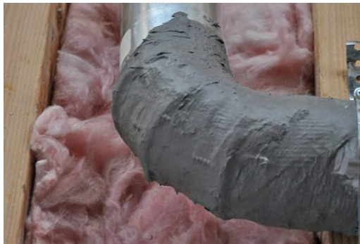
Apply UL 181 mastic or pressure sensitive tapes to seal joint
