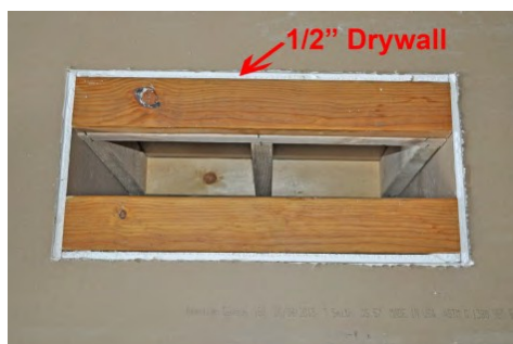
Clear area of debris and insulation in preparation for work
