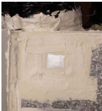
Apply mastic to the seams of the patch.
