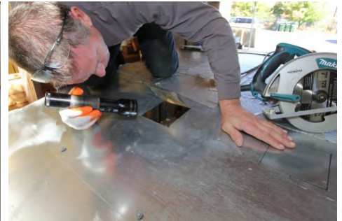
Regardless of access method, visually inspect attic for existing insulation, wiring, flues, obstructions, and hazards
