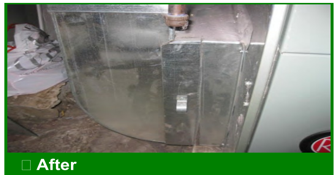
Filter slots should be covered
