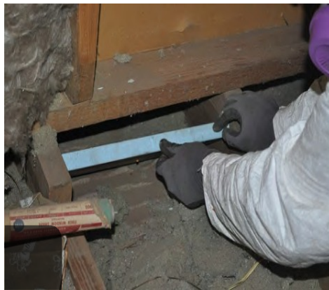
5 Bottom plate is placed in line with interior air barrier
