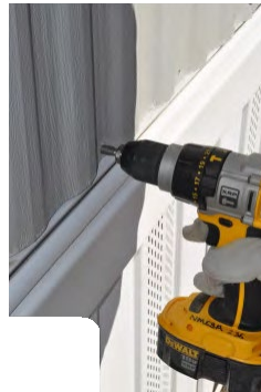
Using new fasteners, reattach paneling
