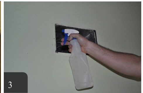
3 Wet the edges of the drywall to ensure a good bond
