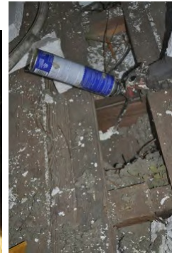
Seal any penetrations
