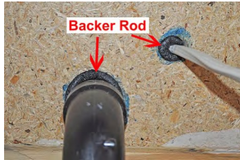
Fill gaps greater than 1/4 inch with backer rod or spray foam
