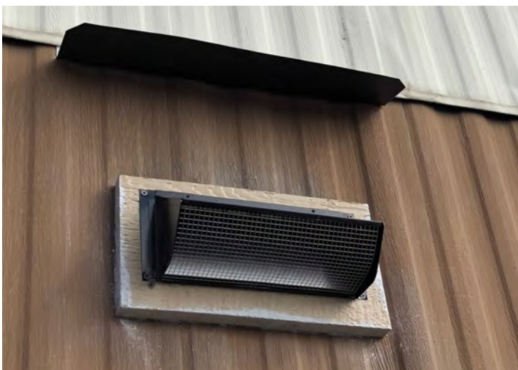
3 1/4 x 9 through wall termination
