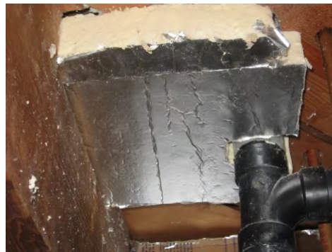
Seal large tub chase using rigid foam then caulk or foam edges
