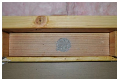
Option 3: Dense pack cavity through fastened wood
