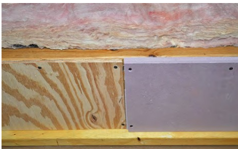
Option 2: Cover face of stud bay with rigid material, like PS or plywood
