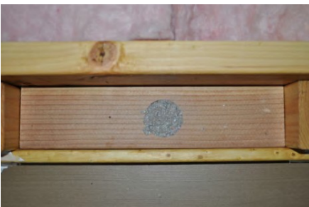
Option 3: Dense pack cavities through fastened wood plate
