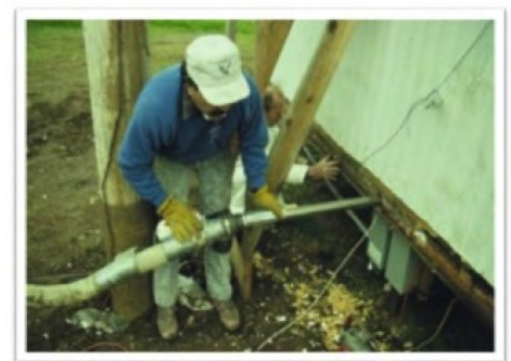
Belly cavity blown by drilling through rim joists.
