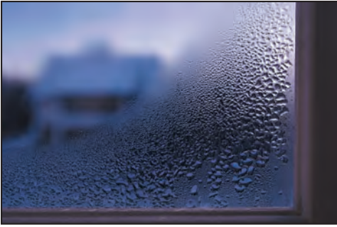
Condensation on the inside of a window-pane.
