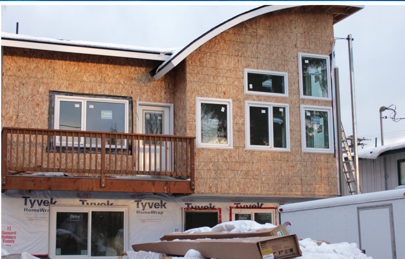
Construction of four-plex on E. Ninth Ave. in Anchorage
