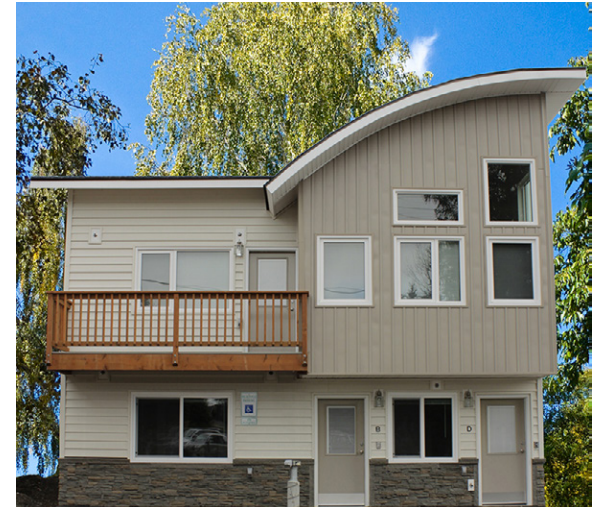
1248 East Ninth Avenue four-plex project in Anchorage.
