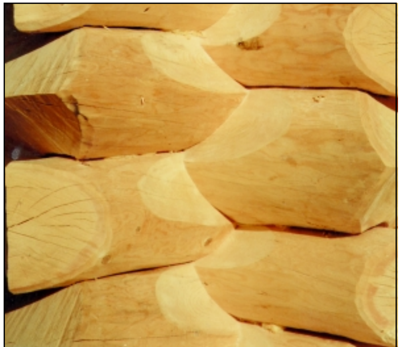
A good modern log home built with a compression-fit saddle notch.
