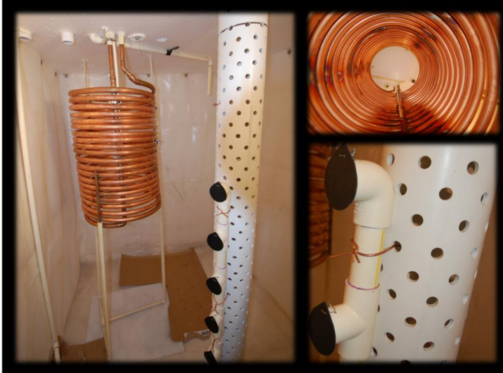
Figure 7: Heat exchangers inside a custom built tank transfer heat to the water in the storage tank. The copper coils transfer heat from the masonry heater, and the white piping transfers heat from the solar thermal panels. The white pipe is perforated to place heated water at a depth in line with the tank's stratification. Photo courtesy of REINA, LLC.
