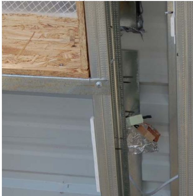
Figure 5. Sensor bundle in mockup wall. Three test sensors were installed just under the window buck, the spot most likely to have water intrusion.
