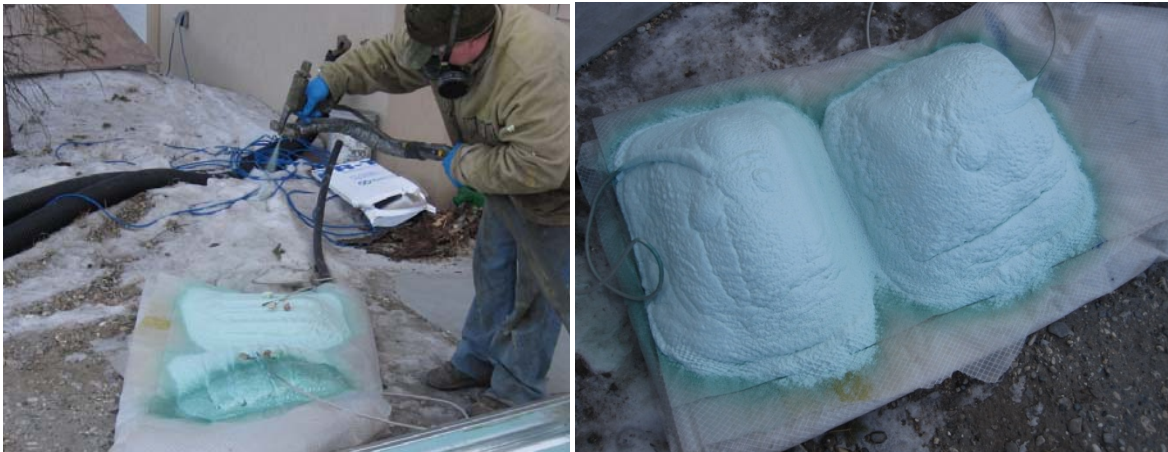
Figure 6. Test pod construction. Each test pods had three test sensors and one temperature sensor within them.
