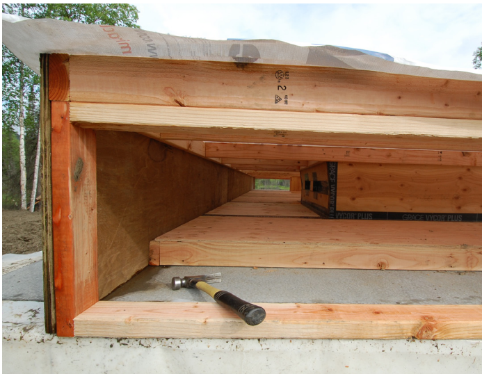
View of the latest version of the wall cavity laying on its side. Bottom is inner structural wall with an air barrier; top is the outer wall.
