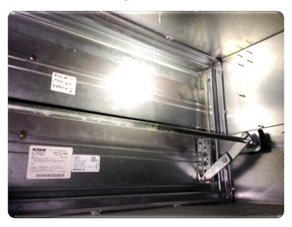
**Before**: The AHU had no minimum air position set point. When the outside temperature was below 55°F, all air was recycled. There was no fresh air
