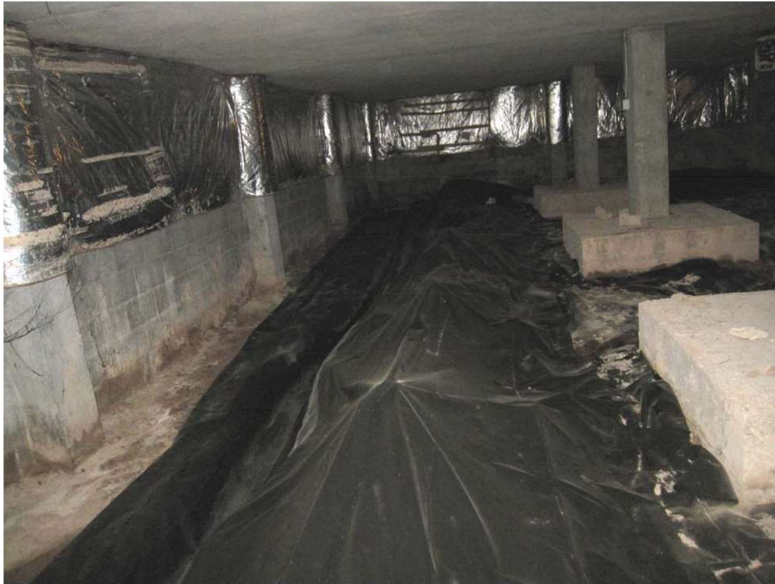
Figure 3 Typical condition at the south wall of the basement – CMU wall; top four feet covered by fiberglass roll insulation; damp footing and lower course; the earthen floor partially covered by black plastic membrane (est. 70% coverage); trench dug near the footing in an effort to direct seepage to sump crocks; concrete interior posts support the concrete floor above.
