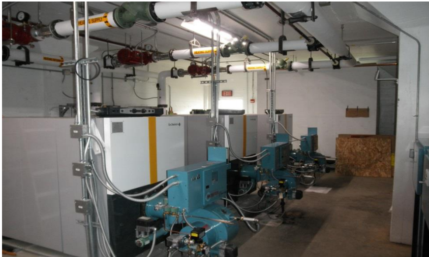
Completed boiler upgrades
