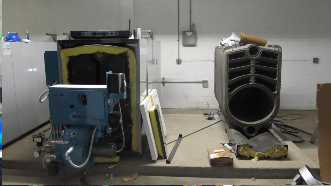
New higher efficiency boilers with DDC controls
