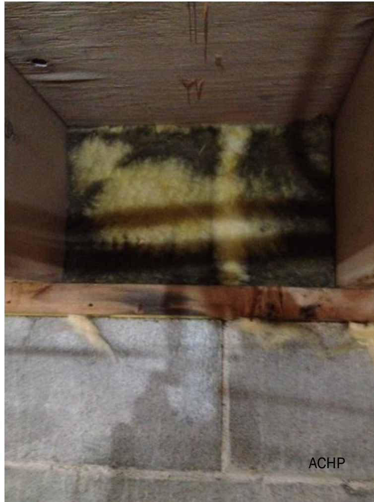
Rim Joist Insulation
