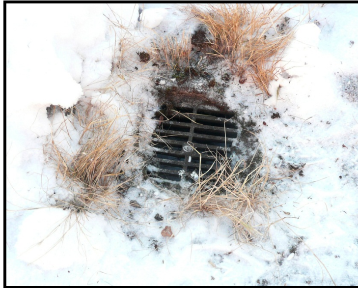
Figure 9: Shrubs and Moss at Upper Level Drain
