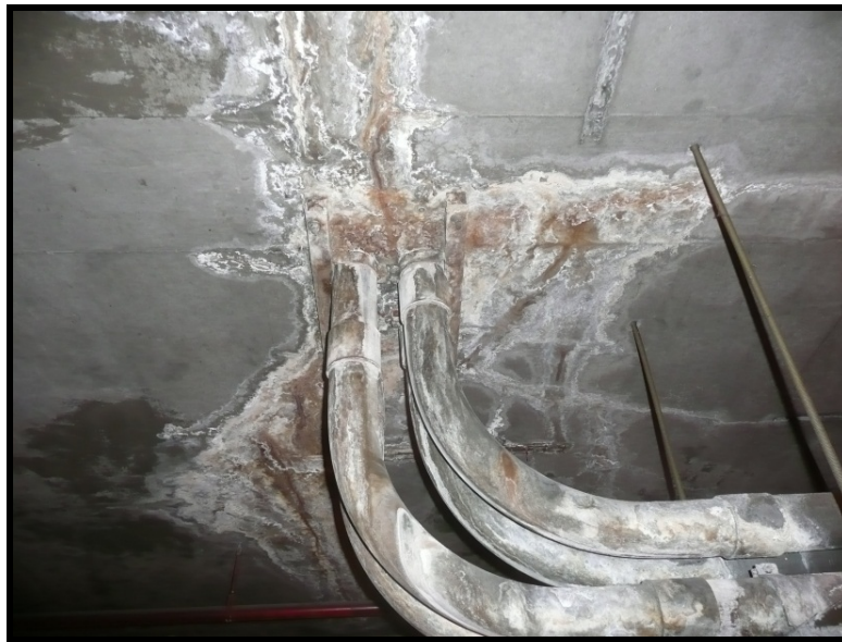
Figure 2: Water Observed at Penetration in Roof Slab
