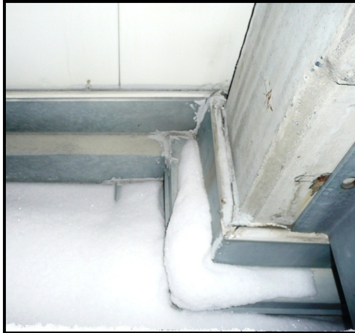
Figure 5: Flashing at Exterior Wall Panel/Concrete Column
