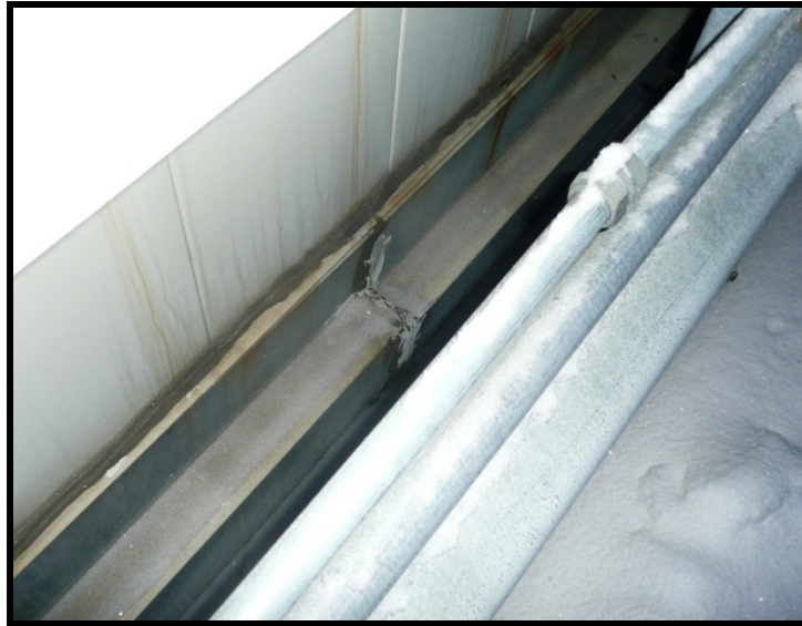
Figure 7: Caulking at Flashing Joints
