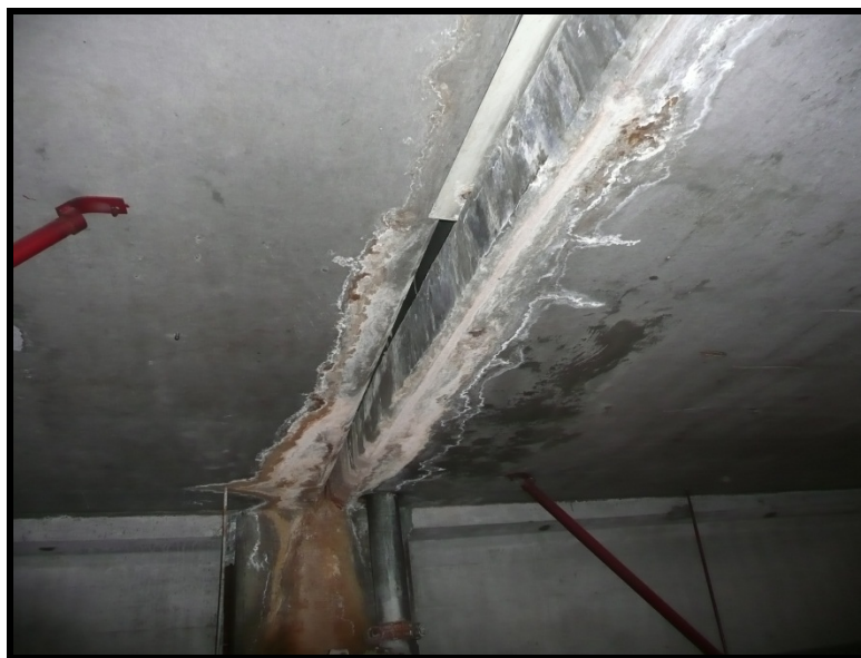
Figure 8: Water Marks Observed Below the Roof Level
