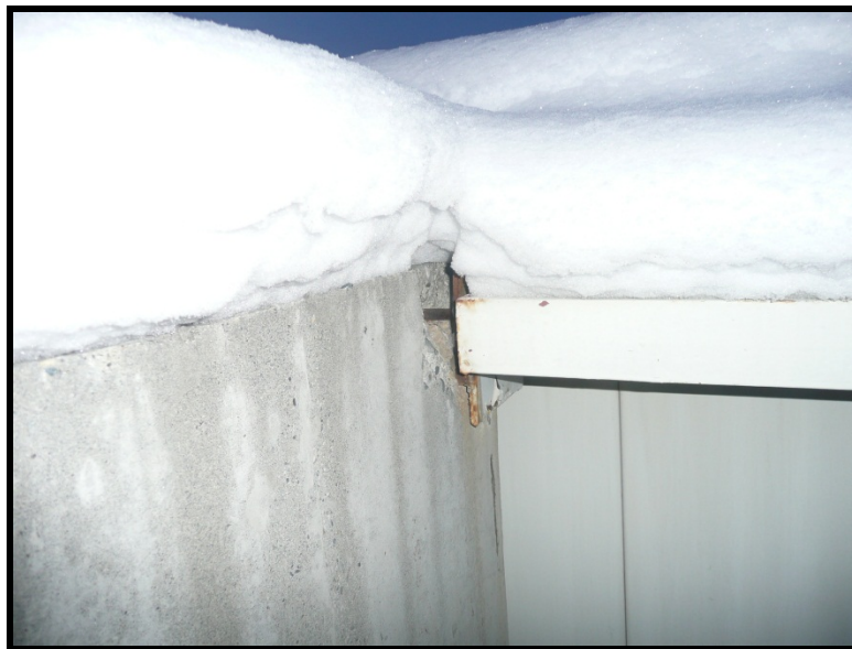
Figure 11: Wind Girt Connection Failure 1
