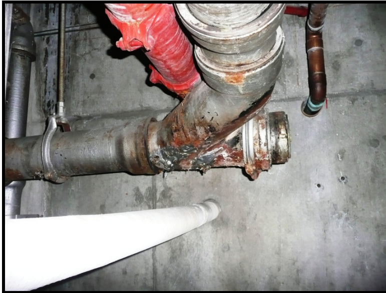
Figure 10: Flexible Caulking Fix on Wye Fitting
