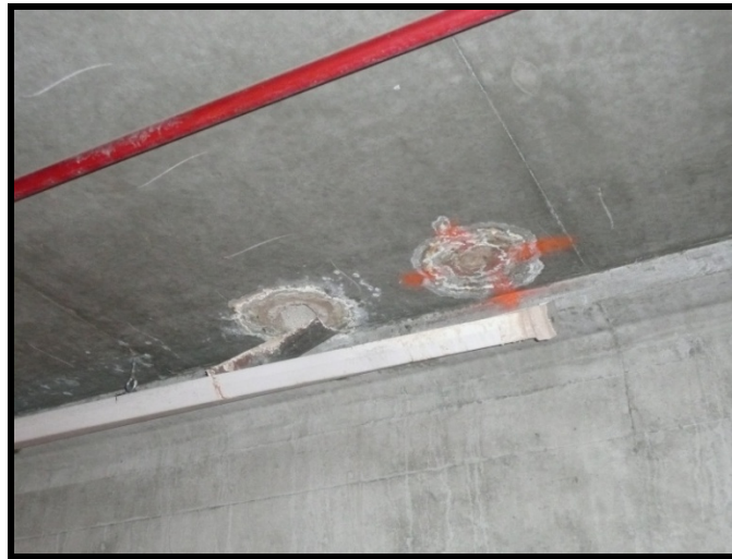
Figure 3: Hole in Structural Slab for Drainage of Between-Slab Moisture
