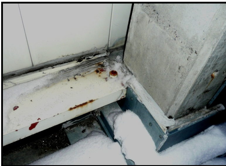
Figure 6: Wind Girt/Flashing
