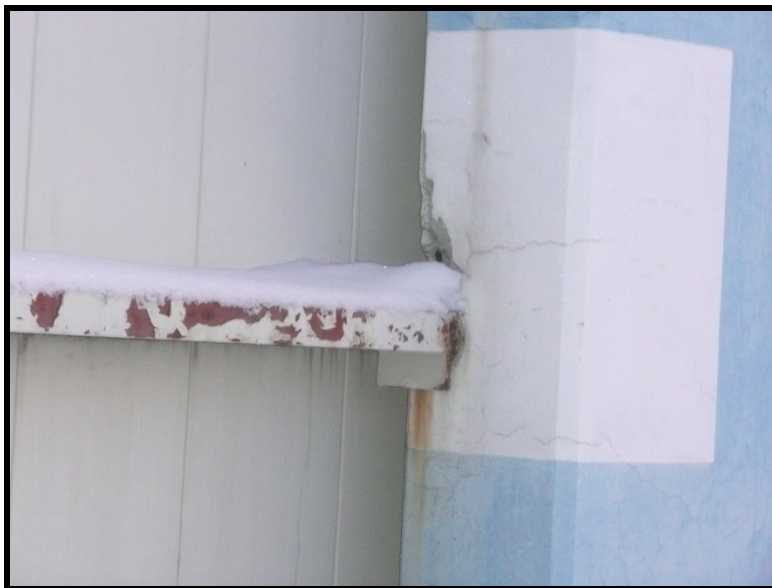
Figure 12: Wind Girt Connection Failure 2
