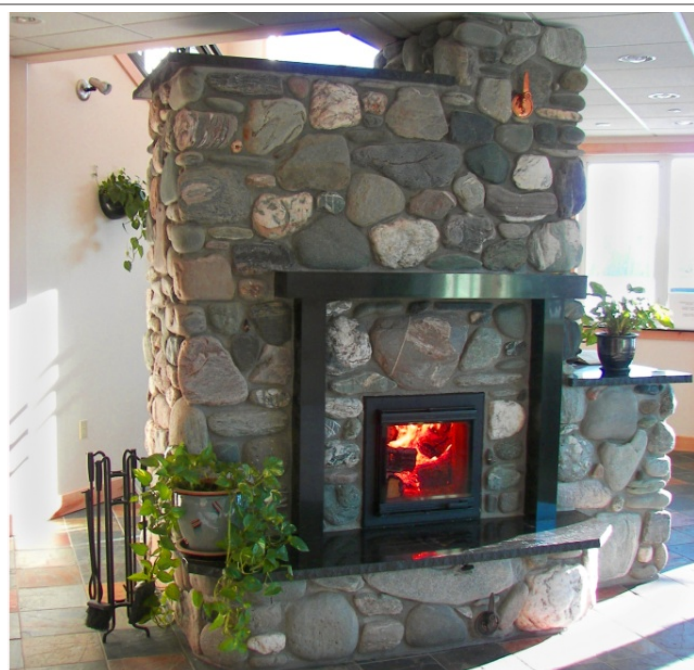
Masonry heaters have a large thermal mass to store and release heat.
