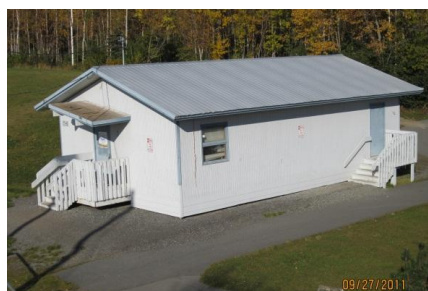
Figure 1: View of Chinook Elementary Relocatable Classroom
