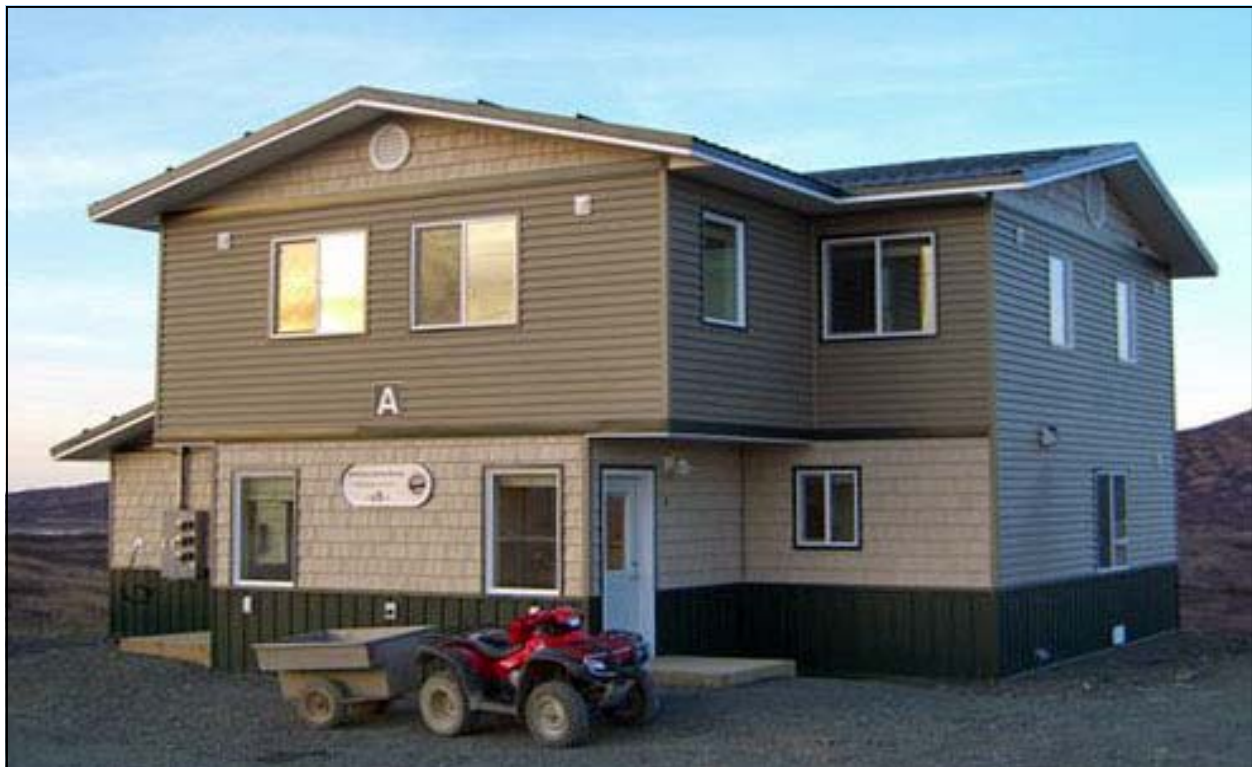
Ten units of teacher housing were constructed in Togiak in 2005, including this duplex.
