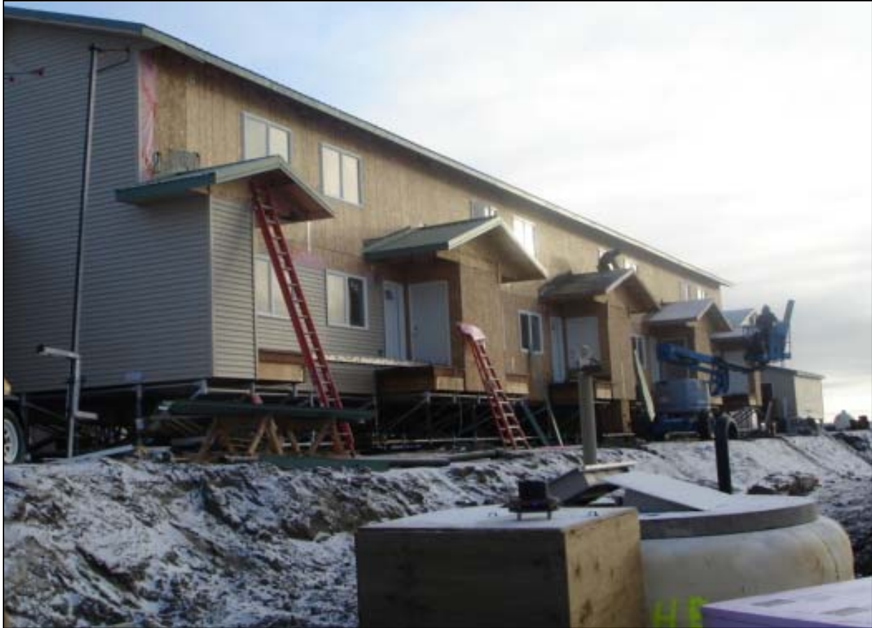
Teacher Housing Units Under Construction in Hooper Bay, 2006.
