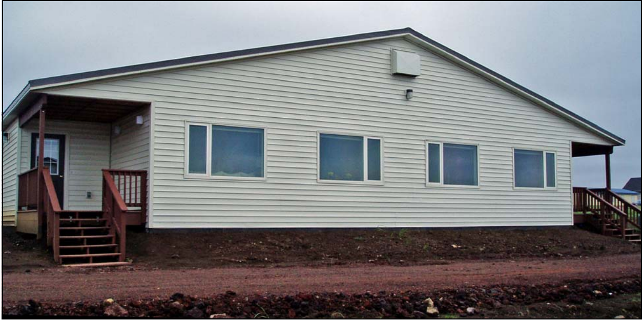
Teacher Housing Duplex constructed in the community of Saint Paul in 2006.
