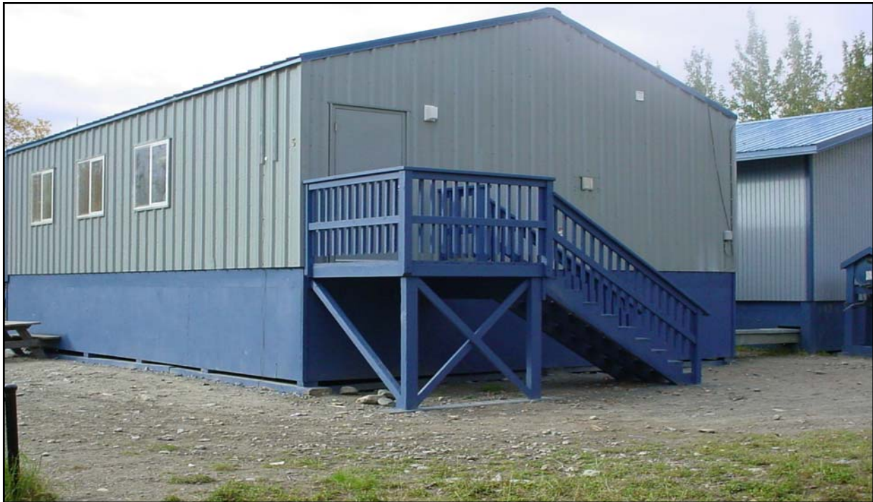
Northwest Arctic Borough converted two relocatables to teacher housing in the Village of Ambler in 2005.
