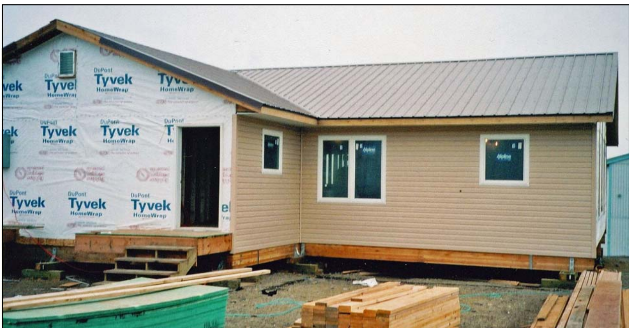
Savoonga Teacher Housing duplex under construction in 2004.
