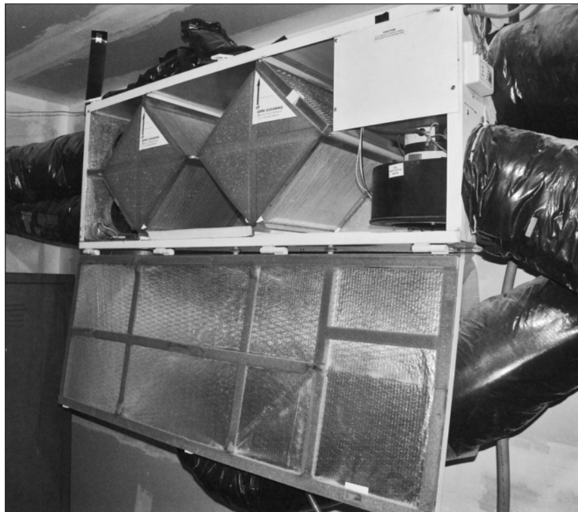
Figure 9.6: A heat-recovery ventilator opened for cleaning and maintenance. Two plate-type heat exchangers are used in this large-capacity model.
