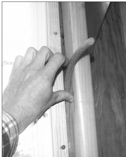
Figure 3.2: Backer rod is a rope-like material made of polyethylene, normally used to seal the space between window and door frames and the rough opening.
