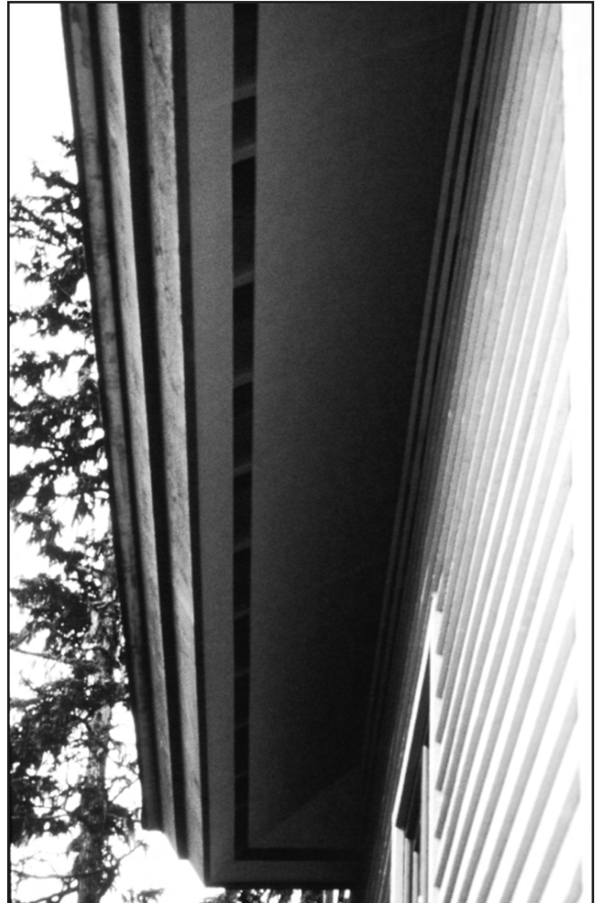
Figure 221. The stand-off furring blocks are attached over the sandwiched screen and original furring. The corner boards have only the original furring underneath them. This gives a nailing base for the corner board and the siding that will butt into the corner board. As the stand-off blocks at the top of the wall are installed, do not install a furring block where the siding is going to marry to the corner board, as this will result in the siding standing out proud of the corner board. The siding is formed, faired, and bent from the corner board plane to the next stud-furring spacer so the air space goes from nothing to the \frac{1}{2} inch space depending on the stud spacing. This holds true when a deck or other mid-wall penetration occurs. Visually it is quite undetectable.
