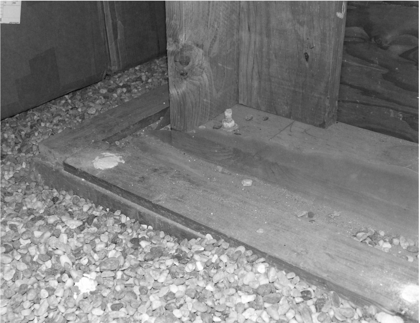
Figure 4.17: A well-constructed foundation with gravel to protect the vapor barrier and boards holding the vapor barrier in place against the footing for a tight seal.
