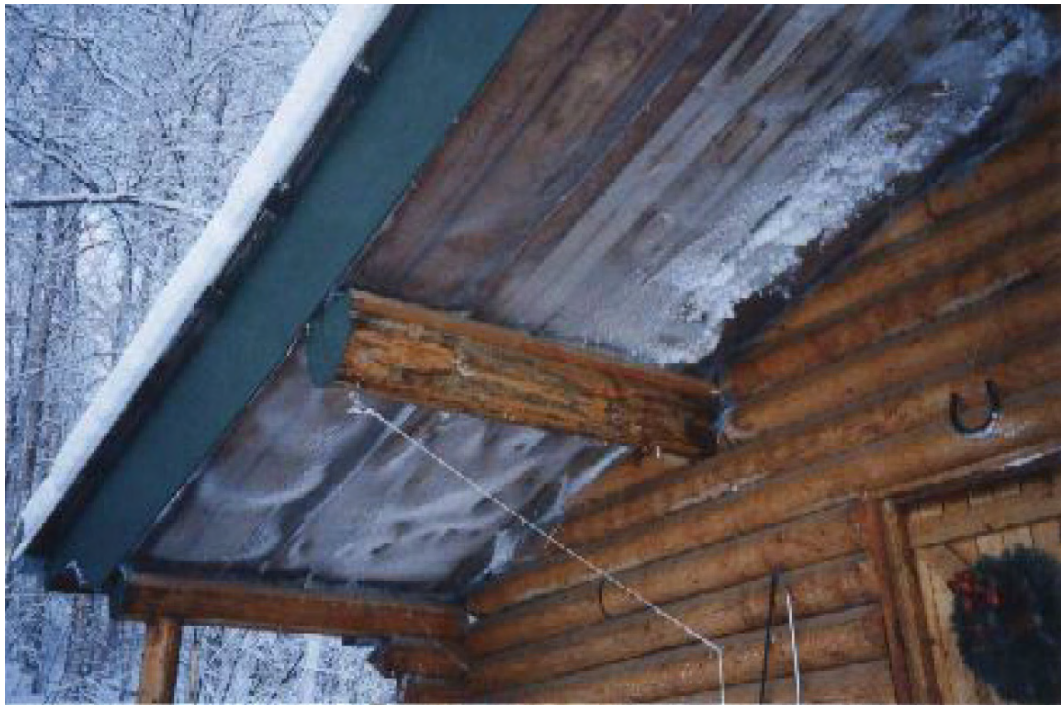
Figure 2.10: This photo shows air leakage at the top of an older log home. Because the air temperature at the time of this photo was -40 degrees F, air leakage is made visible by the accumulating hoarfrost under the eave. The air leakage is normally invisible, and because it is occurring at the ceiling and eaves, is undetected by the occupants. This photo clearly shows that the air leaking out is not only substantial, but it takes moisture with it, which is deposited under the eaves as hoarfrost. Sealing at the roof–ceiling interface and at the gable ends of the roof are very important control measures to ensure this leakage is minimal. Controlling this leakage is not only helpful for good interior humidity but also saves energy by keeping heated air in the house.
