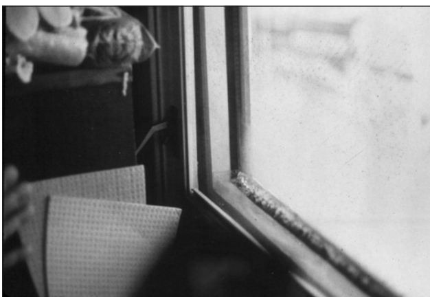
Figure 6.14: Ice accumulation from condensation on the very bottom of a window: the coldest place on any window surface.
