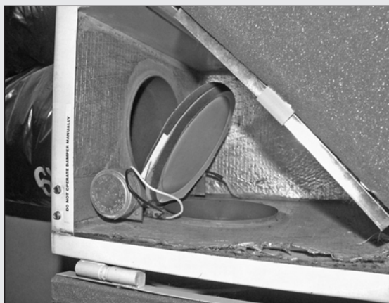
Figure 9.9: This sequence shows a defrost mechanism on an HRV. It operates as a flap valve automatically triggered by temperature to change the source of fresh air for a few minutes. This valve opens ductwork from an indoor source and warm air is run through the heat exchange core to melt accumulated frost from condensation.
