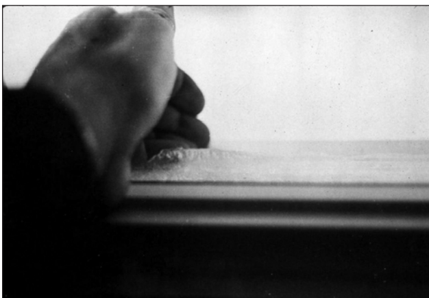
Figure 6.15: Another example of ice accumulation during extreme cold on the bottom of a window pane.
