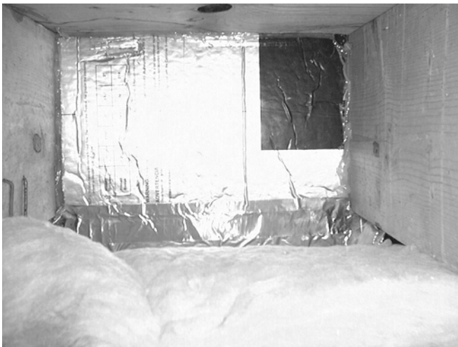
Figure 4.31: Rigid foil-faced foam used to insulate and seal the rim joist. It is caulked to the joists and taped with foil tape to the polyethylene vapor retarder.
