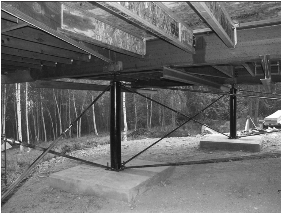
Figure 4.43: The underside of the house in Figure 4.40, showing the concrete pads supporting the posts and the ties holding the posts upright.
