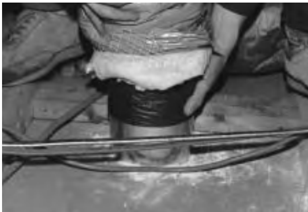
Attaching insulated duct fan ceiling inlet. Ensure gap around duct is sealed where it penetrates the drywall or vapour barrier. Tape ducting to duct fitting.
