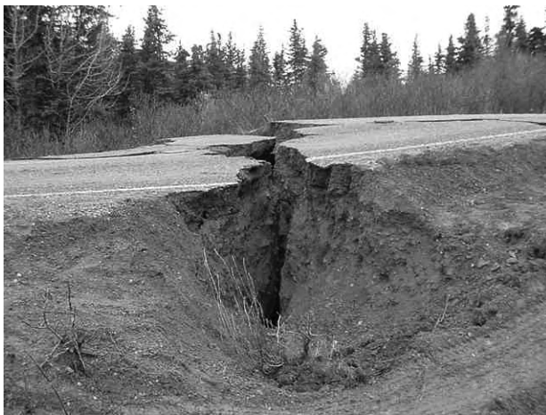
Figure 4.18: A large crack in the highway caused by the Denali Fault earthquake in November 2002.
