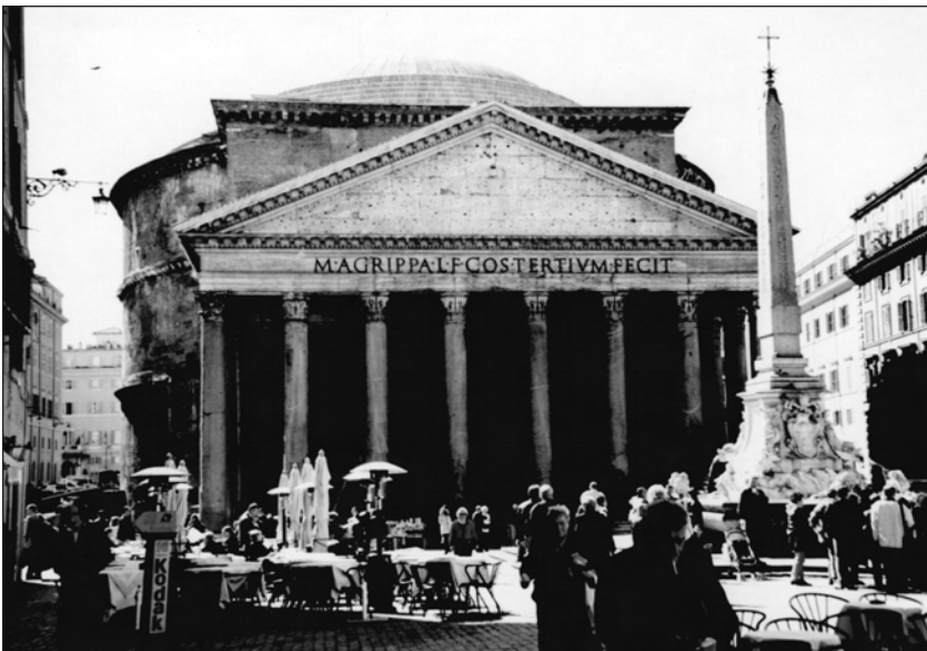
Figure 3.24: At just over 43 meters in diameter, the Roman Pantheon is the largest unreinforced solid concrete dome in the world. The Roman emperor Hadrian ordered it built almost 2,000 years ago. It is still in use today
