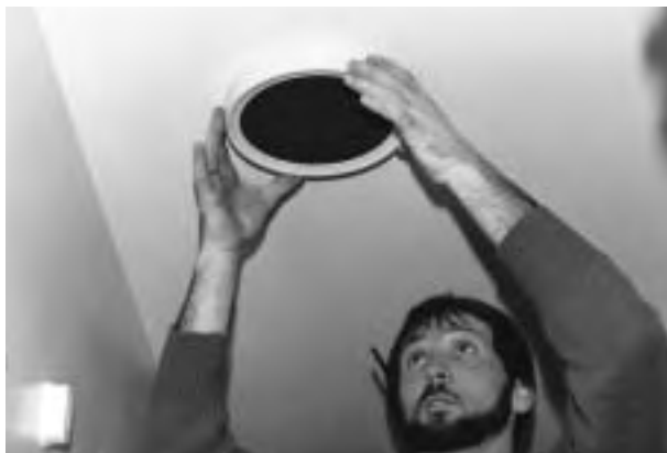
Removeable filter and grille for in-line fan or exhaust vent. Suitable for kitchen and bathrooms.
