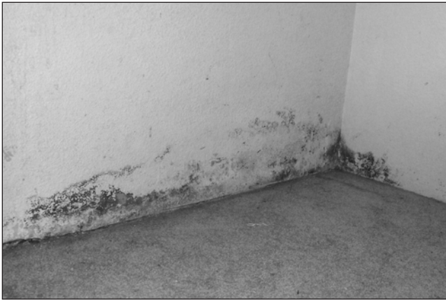
Figure 10.3: Mold on interior walls on an outside corner of the house
