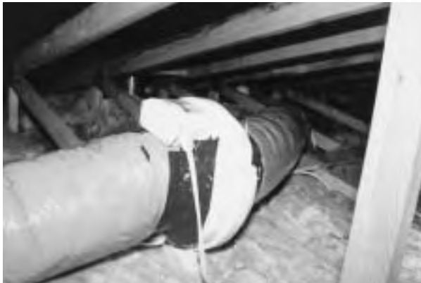
Quality in-line fan unit mounted in an attic. Quiet, capable of continuous operation, and has a high capacity.
