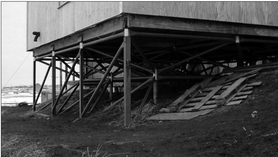
Figure 4.44: A house in Hooper Bay supported by a Triodetics brand frame.
