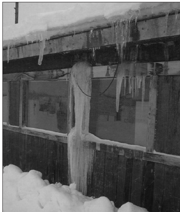
Figure 10.2: Poor candidate for retrofit. This building probably has had ice damage for years and likely has internal damage.
