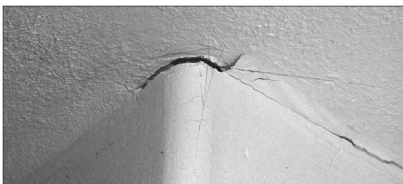
Figure 7.26: Damage caused by roof truss uplift
