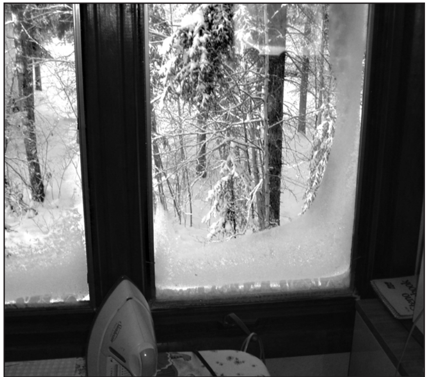
Figure 6.12: Frost has built up between the storm window and the main window. It will eventually melt and cause water damage.
