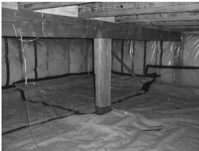
Figure 4.33: A well-sealed crawlspace. Note seams of vapor retarder are sealed with tape.
