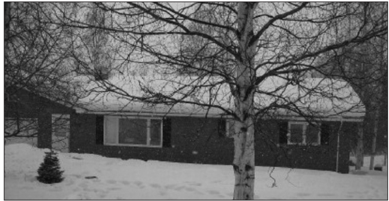
Figure 10.1: A 30-year-old house in Fairbanks that was a good candidate for retrofit. It has a fine foundation; good, well-maintained exterior; and was tested for air leakage and vapor control. It does need new roofing.
