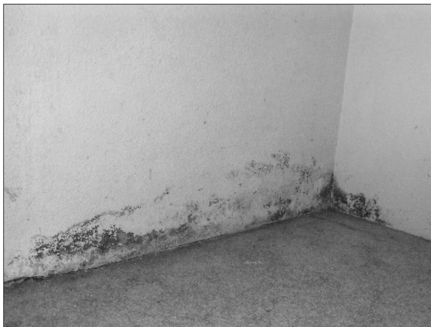
Figure 5.2: Mold on interior walls on an outside corner of the house.
