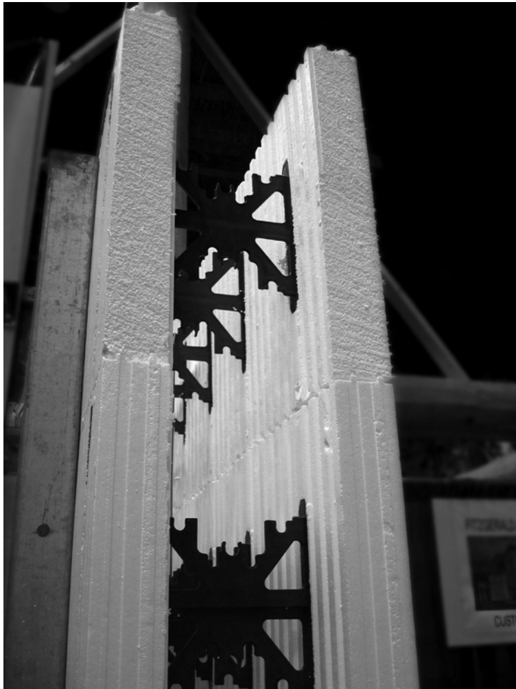
Figure 3. 25: ICFs are rigid plastic foam forms that are filled with reinforced concrete.
