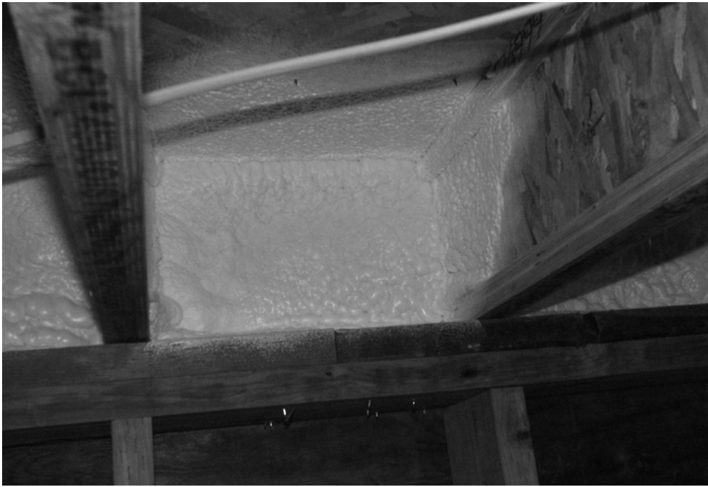
Figure 4.30: Spray urethane foam is used here to insulate and seal the rim joist on an all-weather wood foundation. (Rigid foam was used on the outside of the foundation wall)
