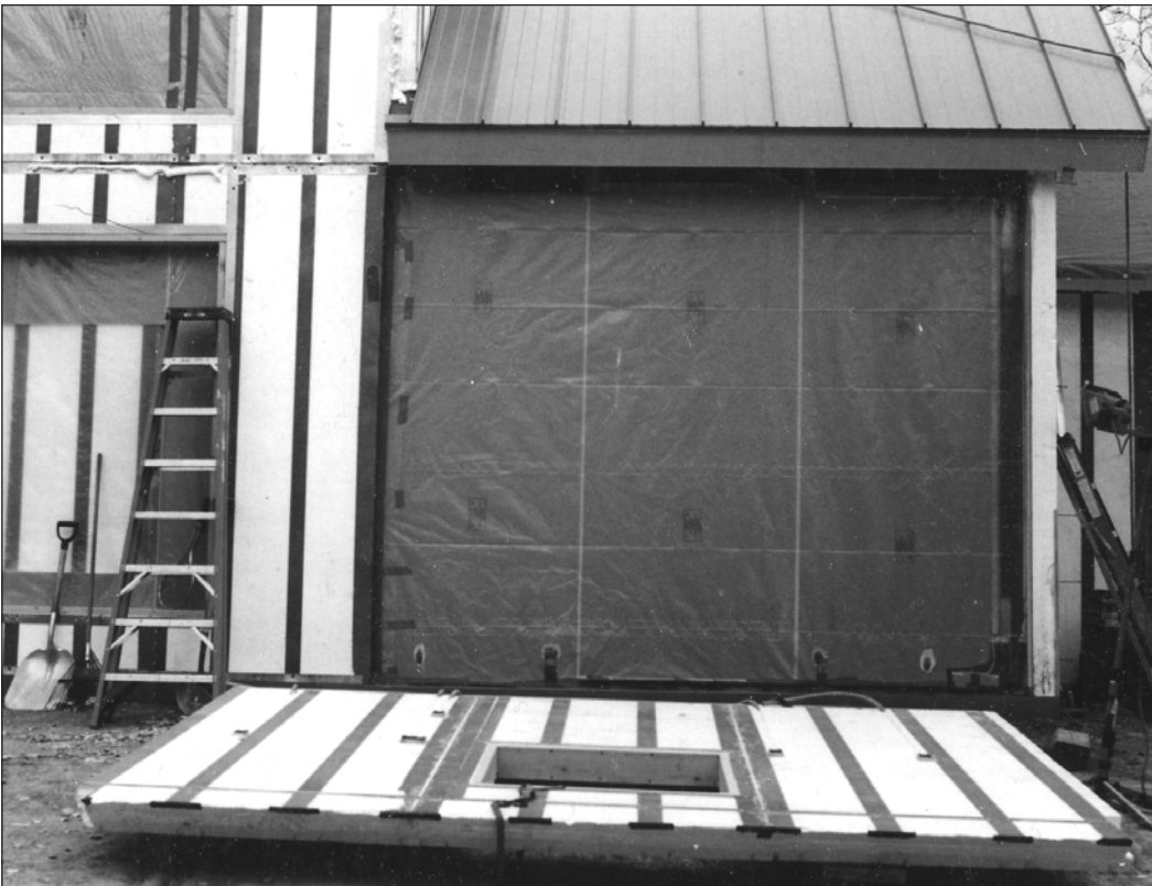
Figure 5.17: This house is being built using structural insulated panels on both walls and roof. The panels are test fitted (top) then laid back on the ground (bottom) and the drywall is placed against the timber frame, then the polyethelene vapor retarder is hung outside of this. Finally the SIPs are replaced. This makes it much easier to install interior drywall against the outside of the timber frame.
