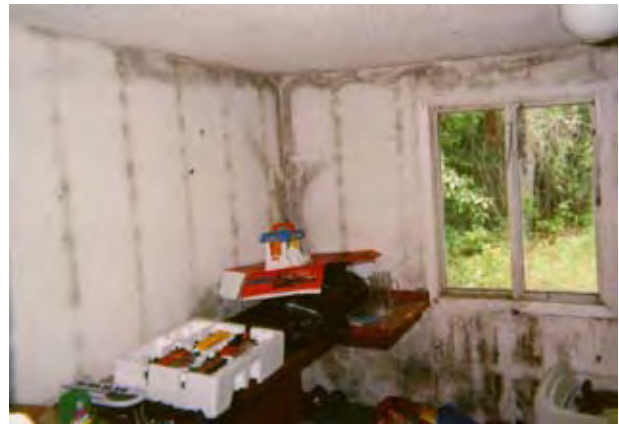
Figure 1. This photo shows several aspects of a house, which is poorly insulated at the studs such that you see condensation and mold not only at the top of the wall where the wall plate is, but also in the corner and at each stud. This is an extreme example of a phenomenon called "ghosting of the studs" where the surface of the wall on the inside of the stud is cooler and therefore condenses out moisture and other vapors on the cool surface first. In the case shown, the problem is fairly horrible with the resulting mold on every cool surface of the inside of the building. Retrofit would solve this by insulating on the exterior or the interior and using good vapor barrier sealing to keep moisture from getting to cold surfaces. The existing condition may also be a result of a fairly tight air seal causing exceedingly high relative humidity levels in the building. Photo by Scott Waterman.
