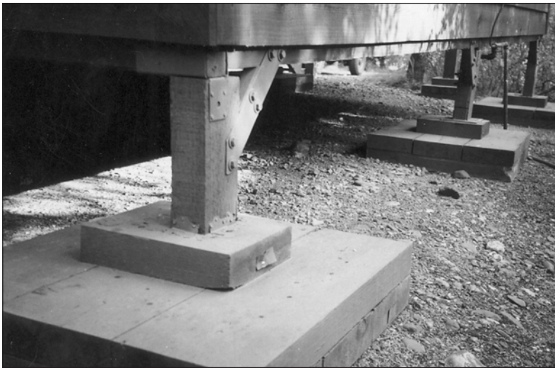
Figure 4.39: This post and pad system has no adjustment and should be used only on stable soils.
