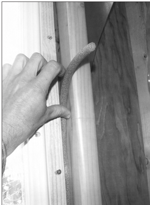
Figure 6.35: Backer rod applied between the window frame and the rough opening.
