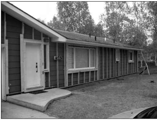
Figure 10.18: A house in the midst of an exterior retrofit. This approach uses narrow wood studs in a wide all-weather wood plate. The top of the wall is attached to the soffit above.
