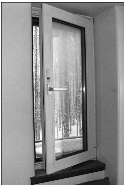
Figure 6.8: A dual-action (tilt-turn) window in the tilt position (top) and in the open or turn position (bottom).
