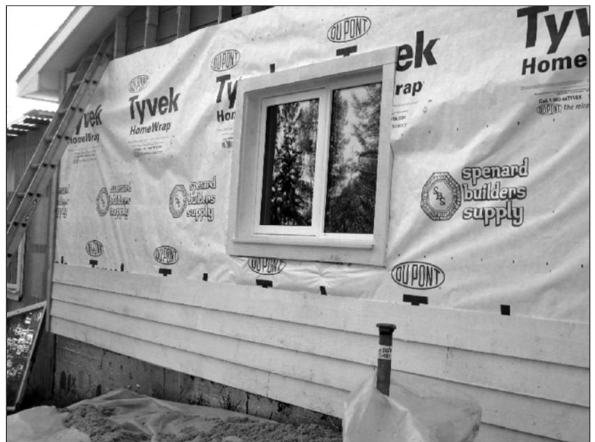
Figure 10.21: This is a view of a side wall with the siding partially placed and the Tyvek installed to the level at which the cellulose is ultimately blown in.
