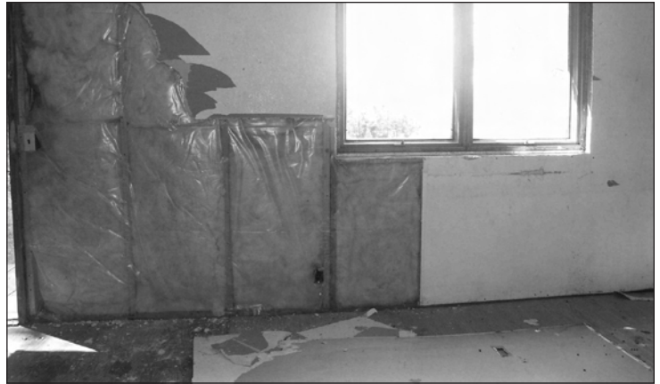
Figure 10.4: Opening up this wall reveals a poorly detailed vapor retarder but good dry studs and insulation.
