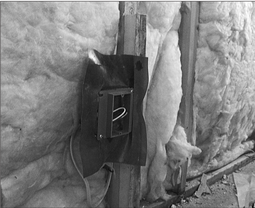
Figure 10.12: A poly pan is used to seal behind an outlet. Foil-backed foam will be installed on the inside of this wall so the outlet is fastened to the furring.
