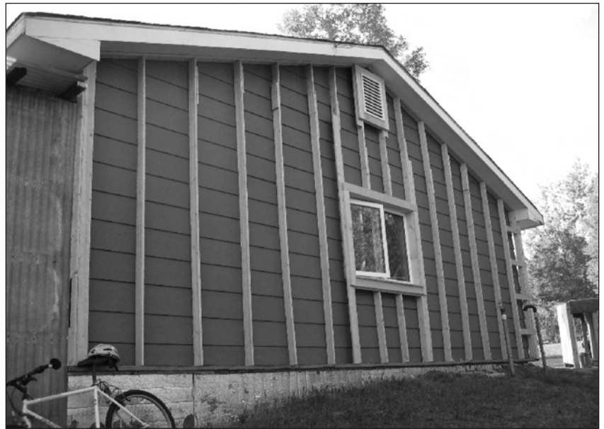
Figure 10.19: This is the east wall of the house before the exterior insulation and finish siding are installed.
