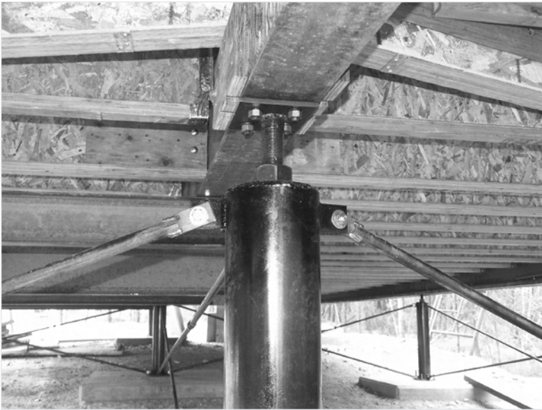
Figure 4.40: This welded steel foundation was custom prefabricated for a building site with discontinuous permafrost and has adjustment to compensate for settling.
