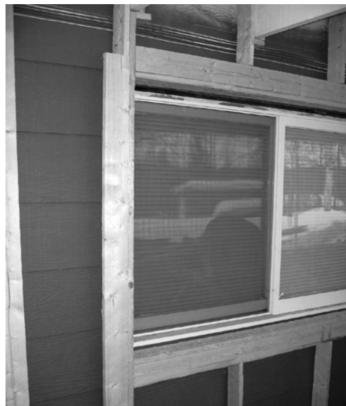
Figure 10.23: A stand-off wall exterior retrofit, showing details around a window opening. In this case the retrofit used a plate at the bottom that was lag-screwed into the original wall plate and then 1 x 4 studs were used as the framing of the new wall.
