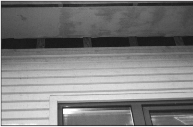
Figure 221. The stand-off furring blocks are attached over the sandwiched screen and original furring. The corner boards have only the original furring underneath them. This gives a nailing base for the corner board and the siding that will butt into the corner board. As the stand-off blocks at the top of the wall are installed, do not install a furring block where the siding is going to marry to the corner board, as this will result in the siding standing out proud of the corner board. The siding is formed, faired, and bent from the corner board plane to the next stud-furring spacer so the air space goes from nothing to the \frac{1}{2} inch space depending on the stud spacing. This holds true when a deck or other mid-wall penetration occurs. Visually it is quite undetectable.
