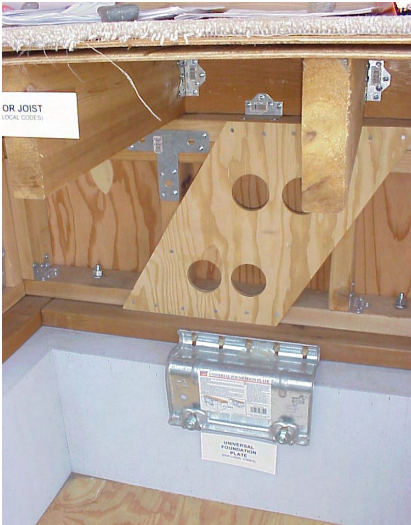
Figure 4.20: A model layout of a foundation with seismic anchors and connectors. This model is used by FEMA to demonstrate materials and examples of seismic reinforced foundation and house design.
