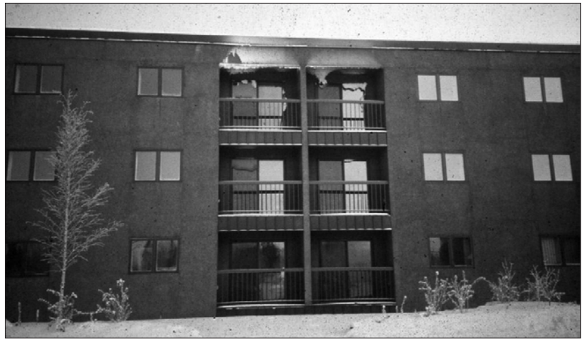
Figure 6.18: This photo shows frost from leaky windows on the top story, while the first and second stories are less frosty.
