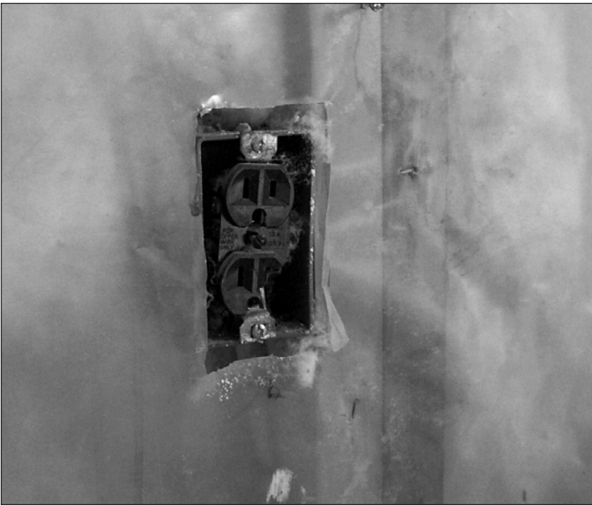
Figure 10.11: A prime site for air leakage around an outlet where the vapor retarder is not sealed.
