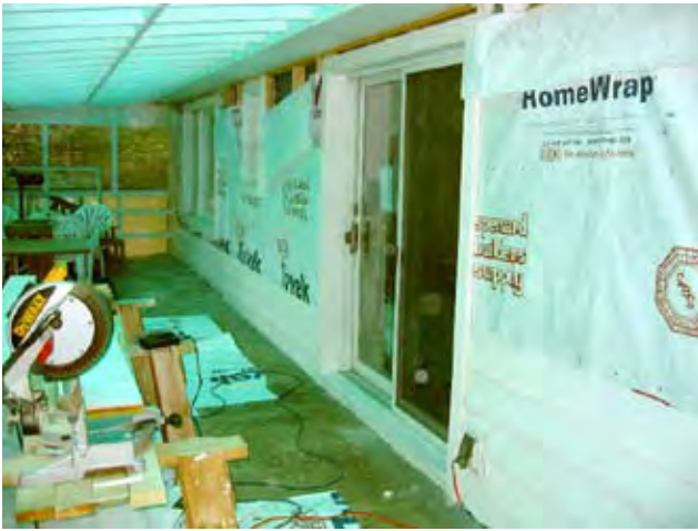
Figure 3. Shows another detail of the author's home in the final retrofit stages. The wall is being covered on the exterior with Tyvek® homewrap and the siding then installed such that cellulose insulation can be sprayed in the wall cavities and below the windows as the siding is attached. The finished wall is then sealed and the insulation is contained by the Tyvek® on the exterior. This system worked extremely well but it only worked well because the new window openings were sealed with foam sealant and the vapor barrier caulked to the inside of the window frame. The vapor barrier itself was of good quality, and had the confidence of the retrofit team that it did indeed stop most of the moisture at the inside wall. These two photographs (Figures 2 and 3) are indications of one way to amply retrofit a wall of a house to achieve a good result. The wall shown in Figure 3 resulted in approximately an R-27 wall when it was originally about R-11. This nearly tripled the insulating value of the wall.
