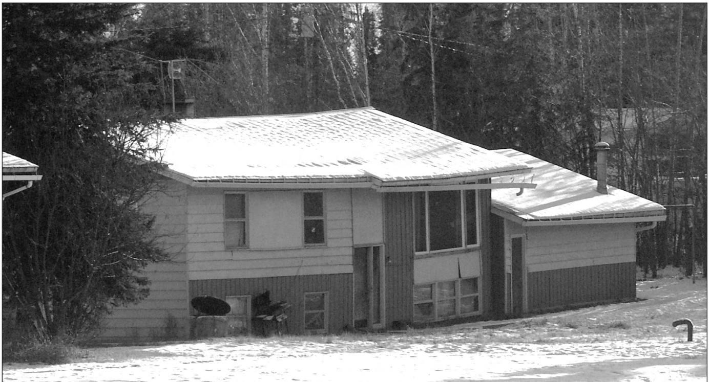
Figure 4.1: This house was built with a conventional foundation on permafrost or an ice lens.
