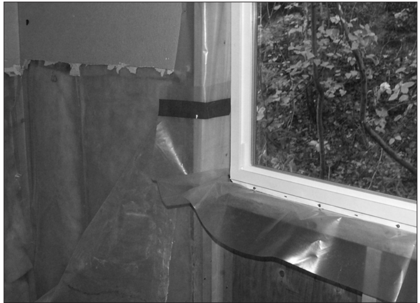
Figure 10.14: A replacement window with the vapor retarder ready to tie into the wall vapor retarder.
