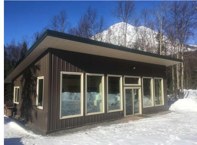
6 Star home built by Jon James Construction
